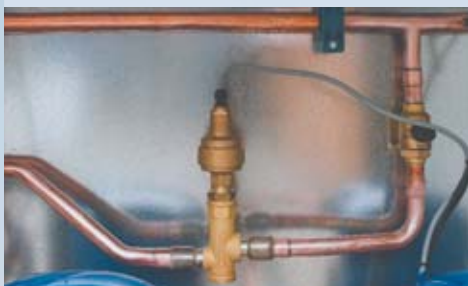
Electronic hot gas by-pass valve
