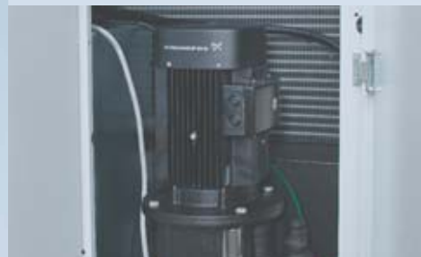
Multi-impeller stainless steel centrifugal pump
